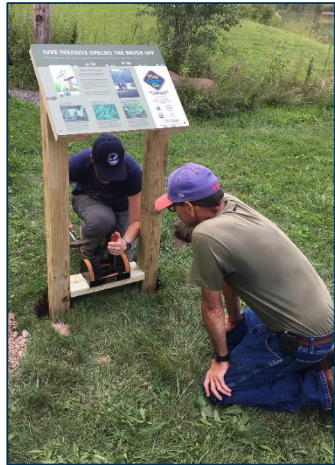
Boot Brush Station installation at Trestle Park.
