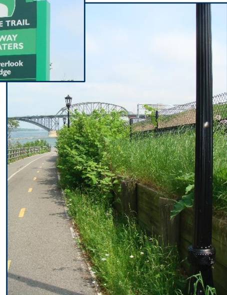
Primary targets for removal along the Riverwalk included knotweed, Phragmites and wild parsnip.
