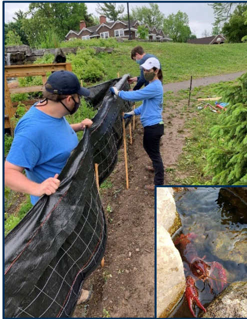
The Crew installed a fence at the Park School on June 3, 2021, to contain the red swamp crayfish population within the pond.
