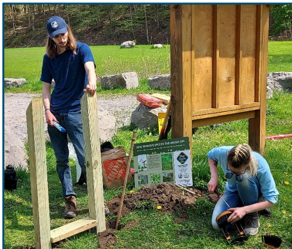
WNY PRISM Crew assisted with the installation of a boot brush station at Cazenovia Creek FWMA.
